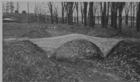
The concrete bridges at Woodmont are attractive, permanent and, best of all, cost but six dollars for material.
