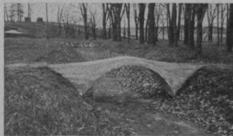
The concrete bridges at Woodmont are attractive, permanent and, best of all, cost but six dollars for material.
