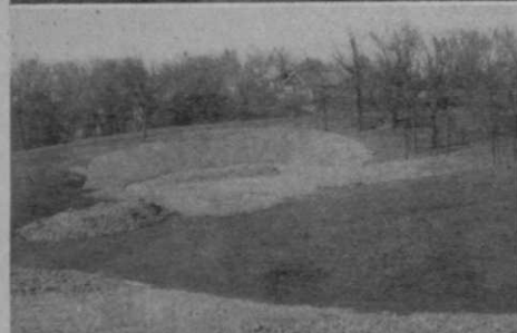
Three views of Des Moines' new muni course. Over 350 workers have been employed at one time on this job.
