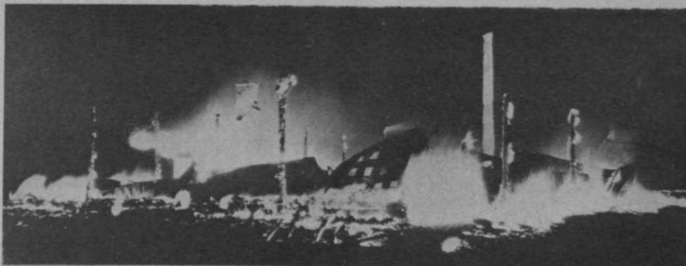
When a clubhouse burns, the loss is generally complete.
