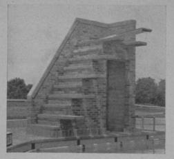
The high dive, with diving elevations at two-foot intervals, is constructed entirely of brick and concrete with the exception of course, of the top springboard. Water is 9 feet deep at this point.
