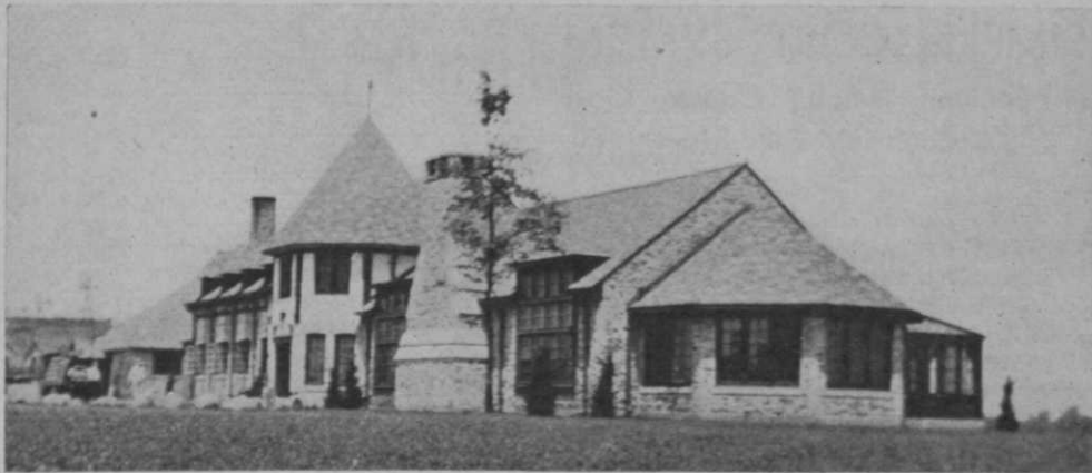
North Hills C. C., Menomonee Falls, Wisc., is one of the leading clubs of the Milwaukee district. Here is a view of its attractive and well-designed clubhouse.
