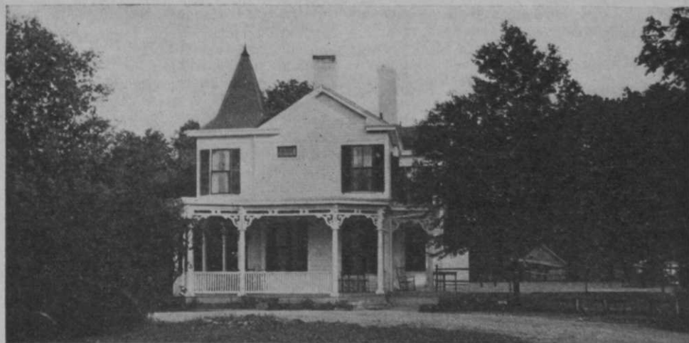
Terrace Park remodelled this residence into a satisfactory clubhouse by adding the low-lying locker-room addition at the right. The roof of the locker-room serves as an outdoor dance platform.
