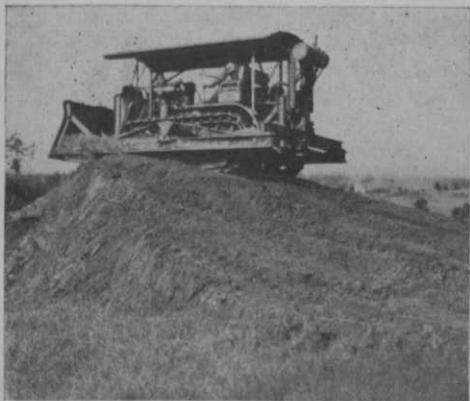
A typical Mackenzie green is swiftly built by Caterpillar
