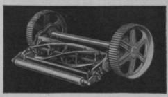
Using the most powerful frame, double sets of tempered steel cut gears in oil tight cases, Timken Bearings—it lasts longer.
