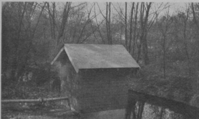
This pumphouse, on the banks of Kyte Creek, cost only $250 to build.
