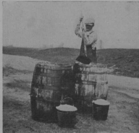
Mixing the iron sulphate calls for exact adherence to the directions. Have dependable men on this job.
