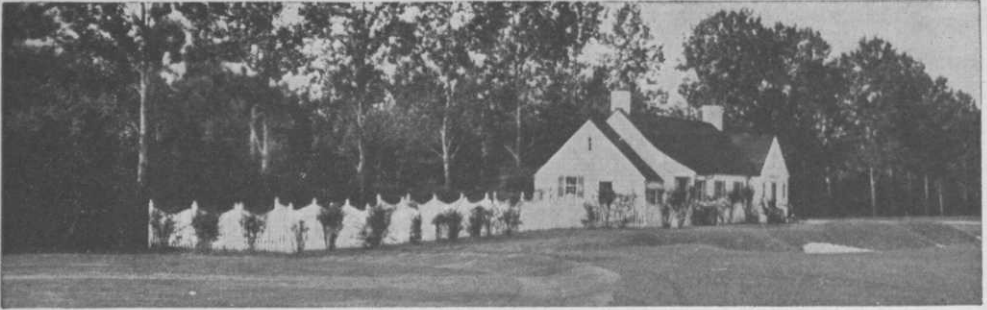
This de luxe building and yard is for the caddies at the Crescent Athletic Club's new layout at Huntington, L. I.
