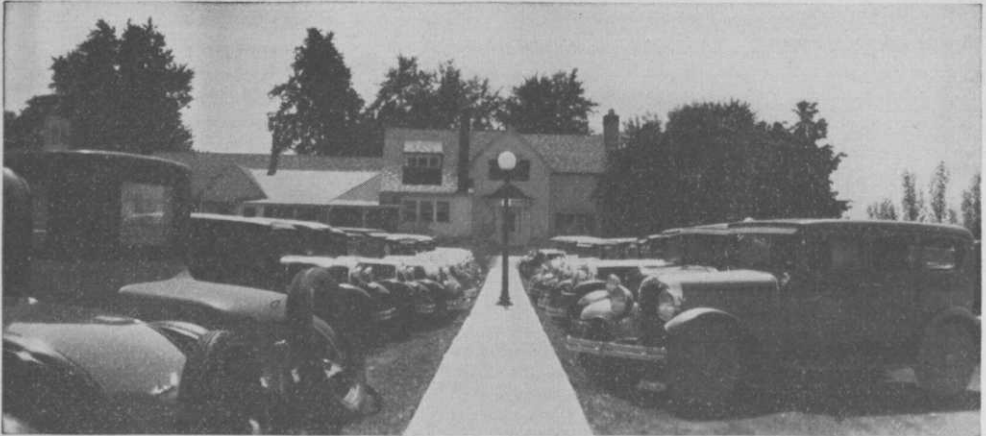
At Meridian Hills C. C. (Indianapolis distr.) a concrete walk in the center of the parking space and leading to a clubhouse door, is a thoughtful handling of a perplexing problem. Especially on rainy party nights the golf club automobile parking stands out as one of the sore spots of most plants. The Meridian Hills installation suggests that elevated concrete walks, possibly with posts for canvas canopies during rains, might be laid out in a manner that would make parking far more convenient.
