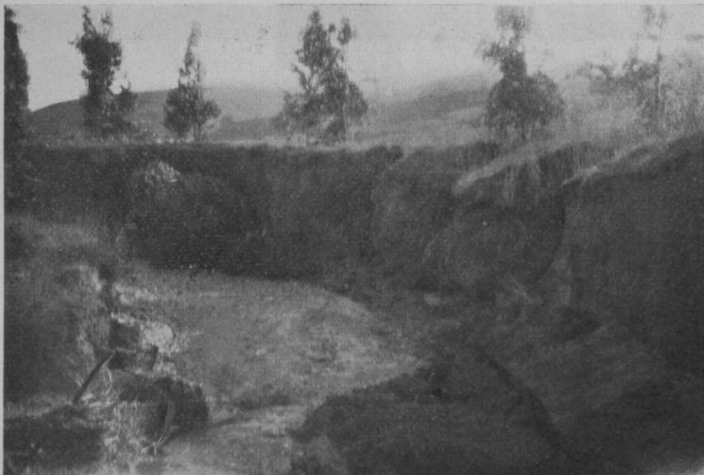
How storm waters destroy in California. Newly eroded banks on the course of the Hillcrest C. C. of Los Angeles.
