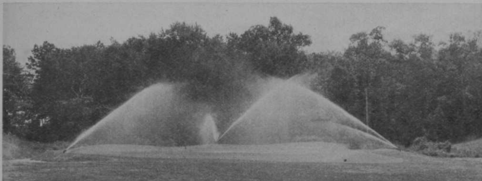
Hoseless irrigation for the putting green of irregular contour. The three sprinklers are permanently installed, and controlled by one valve.
