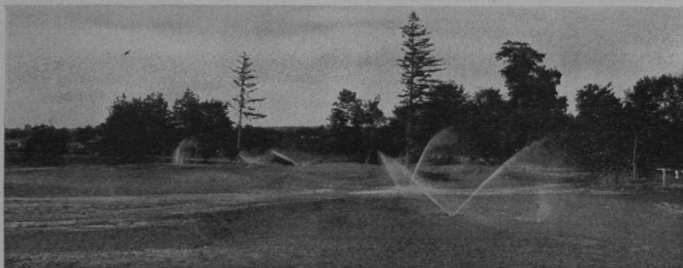
Concealed tee sprinklers in "mow-over" tees at University of Michigan's new golf course
