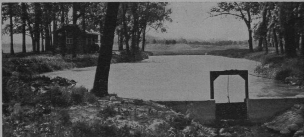
Midlothian C. C. (Chicago district) has a water system that combines deep wells, a stream and this reservoir site. The pumphouse shown has automatic pressure control apparatus as a feature
