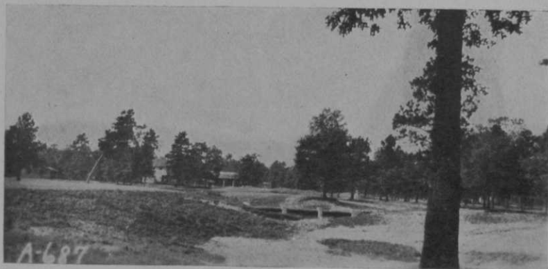
After: Backfill is completed. Note improved appearance.
