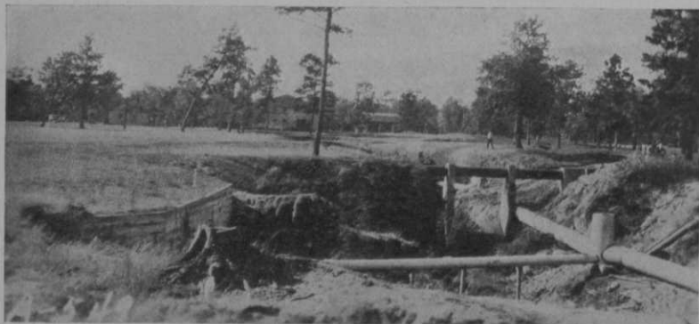
Before: Pipe in place and backfill in progress.
