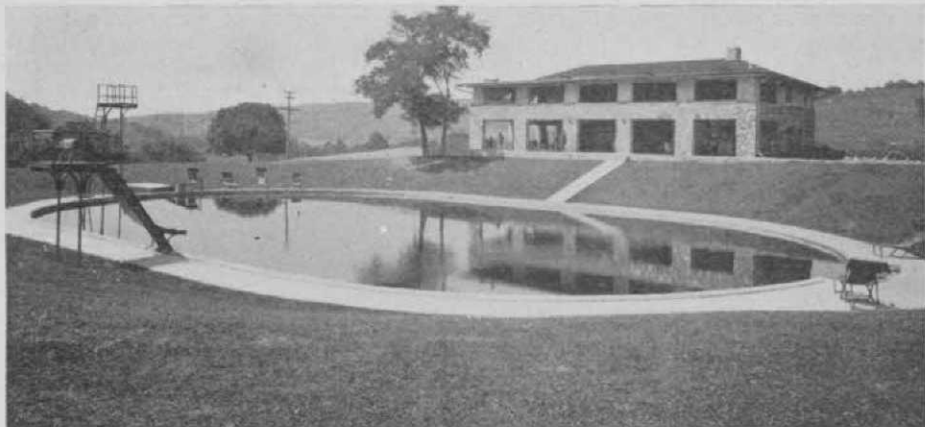
The Juniata Valley C. C. swimming pool is built on a plateau sloping away from the clubhouse, so excavation and fill costs were cut down
