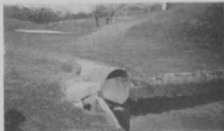
A brook at an inconvenient place was carried under a fairway into a lagoon.
