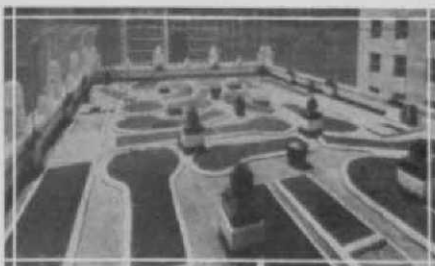
This Shaw course on a Dallas roof was one of the first of the now numerous installations
