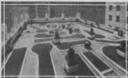
This Shaw course on a Dallas roof was one of the first of the now numerous installations
