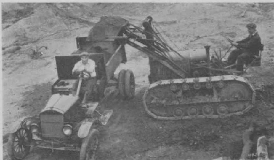
This tractor outfit with scoop and loader is kept busy all through the season, and then some, at Medinah in the Chicago district. It handles material for road and trap maintenance, compost, and is a money—and time—saver on construction jobs.
