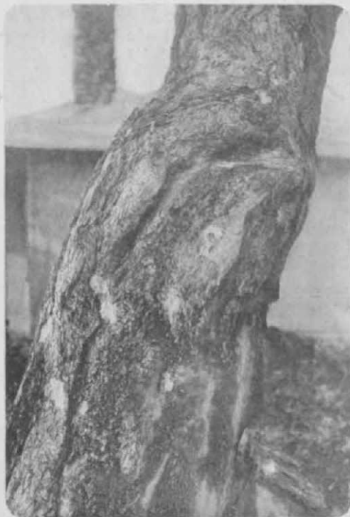
A close-up of the job—the light spots are putty, used in closing up the beetle holes so successfully
