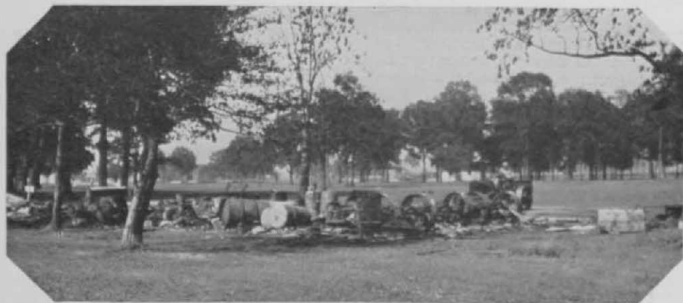
A few days ago this was the site of a fine equipment shed, stocked with $15,000 worth of maintenance machinery and supplies. Just a spark and a night wind, and the result is shown here. Now the club is learning a lot about insurance.
