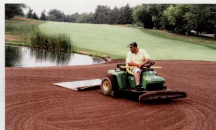
Doing contour adjustments and applying the finish grade.
