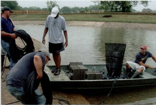
Above: Installation of an aerator fountain.
