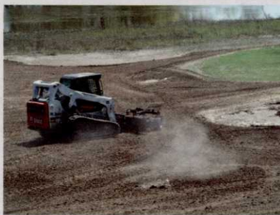
The rebuilding process following the record flooding of 2009 took several months.
