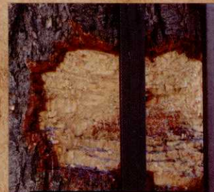
Vandalism at Chambers Bay
