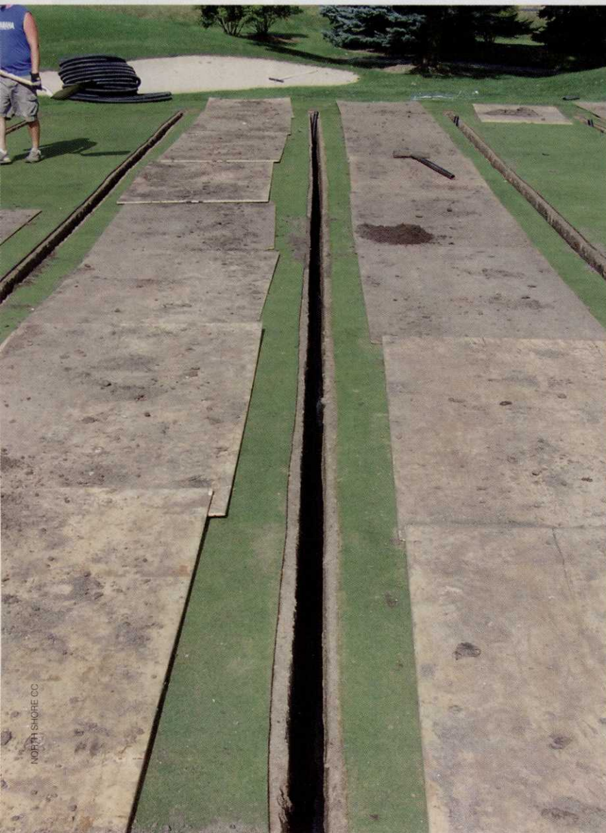
The greens drainage installation project underway at North Shore Country Club.
