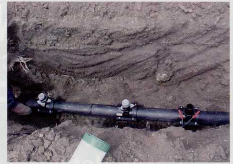
An electro-fused 4-inch by 2-inch saddle.
