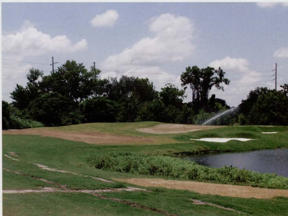
To ensure drainage problems were solved, drain lines were installed every 15 feet through the fairways. Photo: Interlachen Country Club
