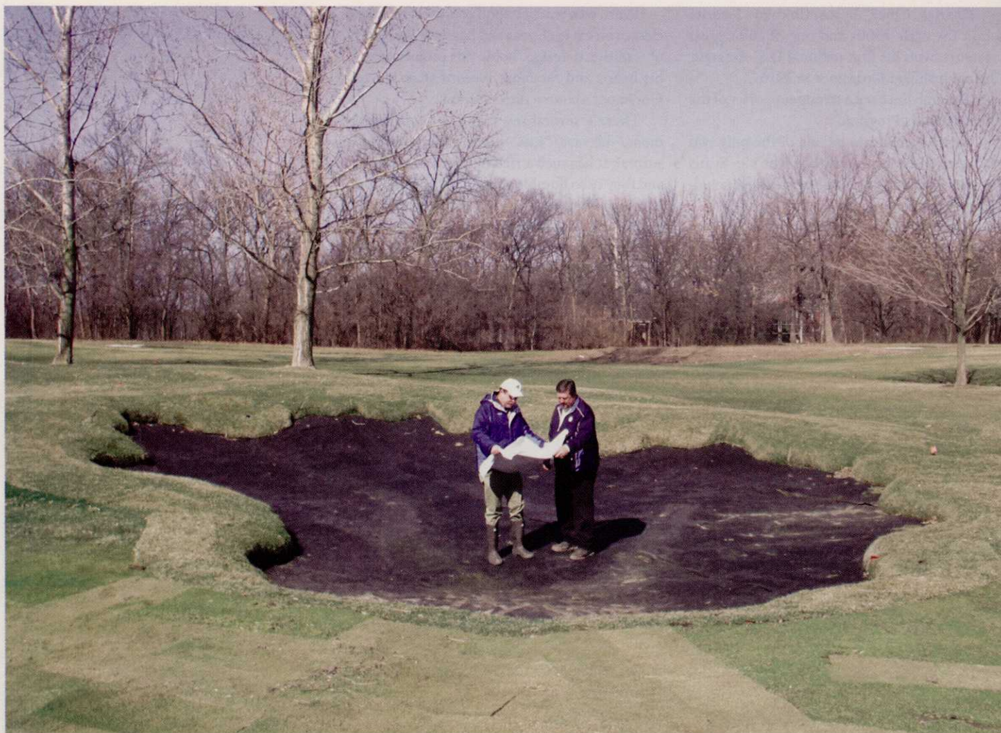
Golf course architect Raymond Hearn and golf course superintendent Robert Lively examine construction plans and a new bunker liner before sand is installed. Photo: Flossmoor Country Club
