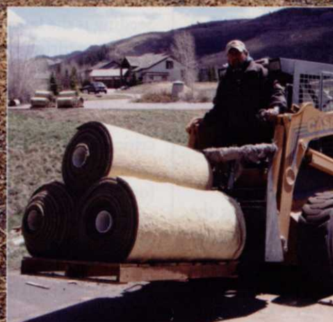
Sprigging is the common method of establishing warm-season grasses, but sodding (inset left) continues to gain popularity with golf course construction. The advent of big roll sod (inset right) has made sodding much faster and easier.
