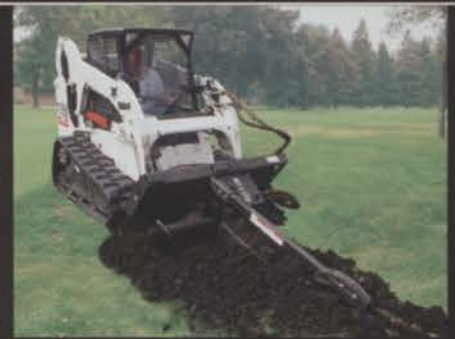
Track loader trenching irrigation line
