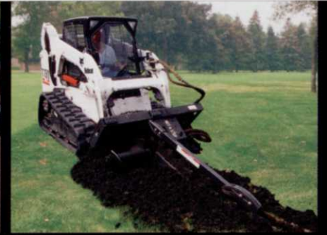
Track loader trenching irrigation line
