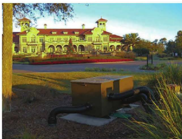
Sub-surface systems move cool air through the root zone to lower soil temperatures. In wet weather, the system removes excess water and increases aeration.
