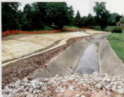
Above: Two images of the new channel next to the old one at Reid Golf Course.
