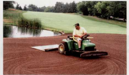
Doing contour adjustments and applying the finish grade.
