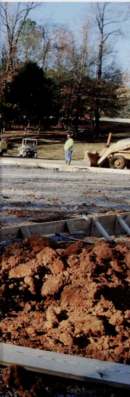
Construction of the new maintenance facility at FarmLinks Golf Club at Pursell Farms in Sylacauga, Ala.
