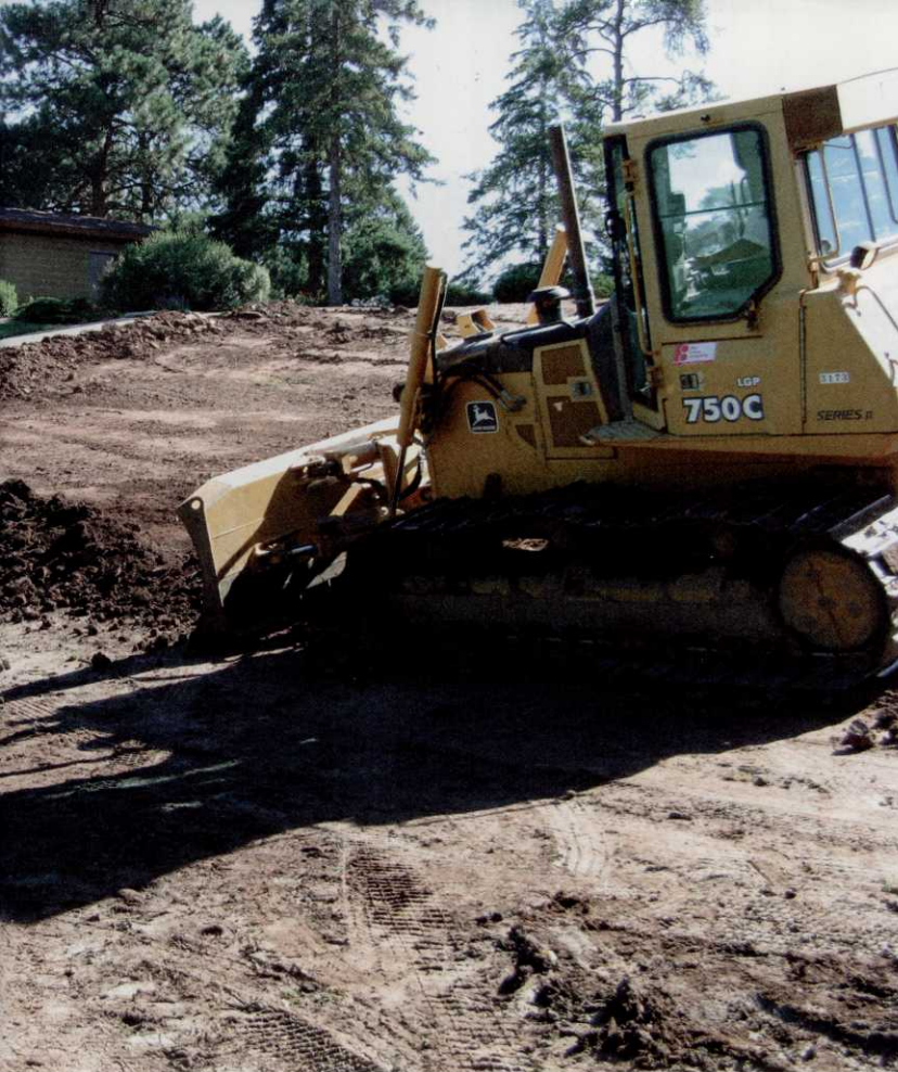
The stripping of the existing topsoil. Inset: A pile of existing mix salvage to be used later on.
