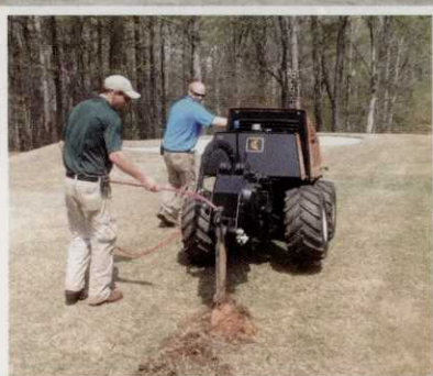
Top Left: Drilling a well at ACC. Above: Adding wire for more stations for greater irrigation efficiency.
