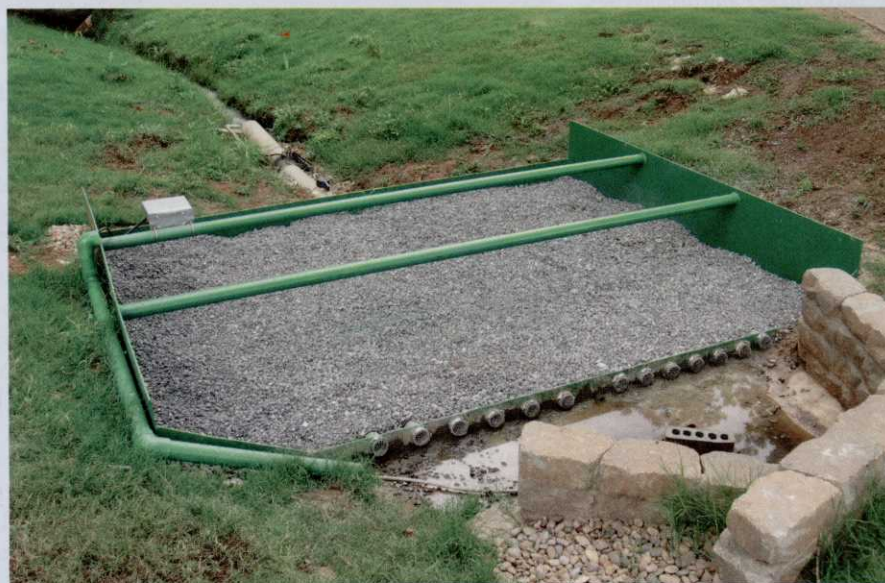
Top: The 150-acre mixed residential and undeveloped watershed in Stillwater, Okla. Right: The completed phosphorus removal structure filled with steel slag.
