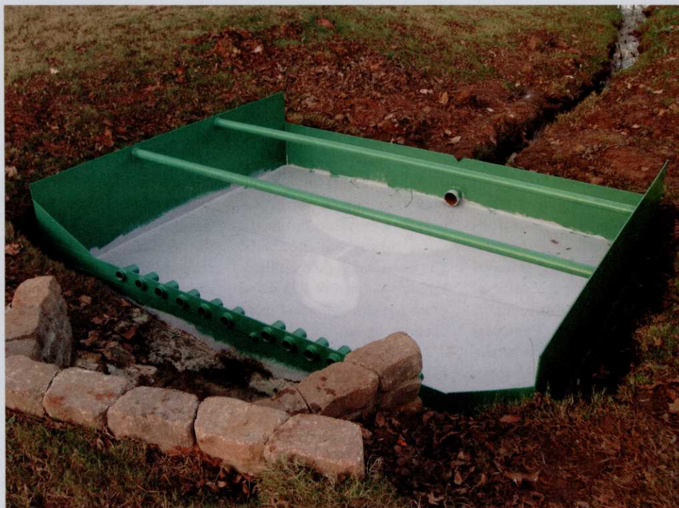
The uncompleted phosphorus removal structure shown during construction.
