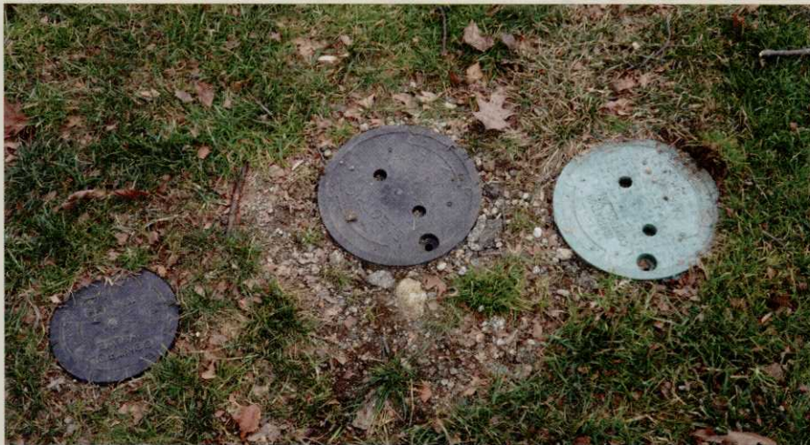
Various valves and splices can be identified by different colors and cover sizes.
