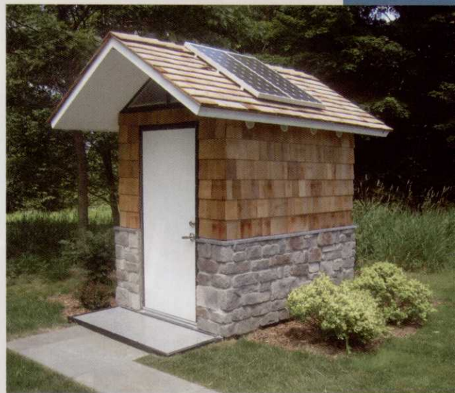
A contractor installed the units' shingle roofs and siding for about $5,000.
