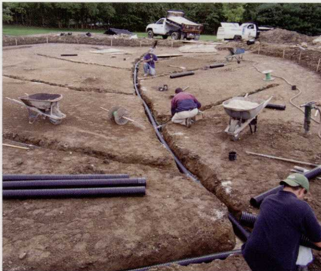
The golf course at Rockrimmon has been through every phase of construction during the past 14 years, from rebuilding greens to USGA specs to improving internal drainage on existing native soil pushup greens (below). Photos: Rockrimmon Country Club
