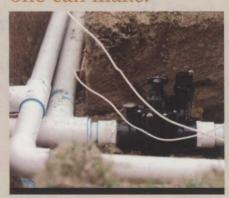
New irrigation system designs also focus more on control flexibility. This allows superintendents to fine tune a system to irrigate different microclimates (such as hills and valleys or shade and sun) much better than designs a decade ago, which focused on minimizing pipe and wire. Better control reduces water use and annoying wet or dry spots, which enhances turf health and play quality.
