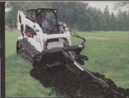
Track loader trenching irrigation line
