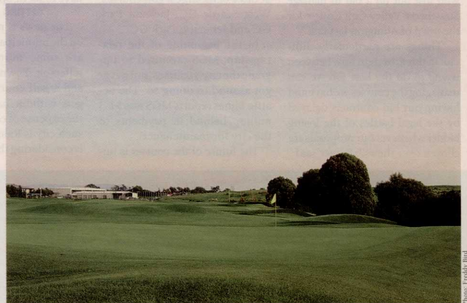
Reconstruction work at the Fred Bliss and Johnny Miller-designed Metropolitan Golf Links included using dredge material from the Port of Oakland to cap an existing landfill.
