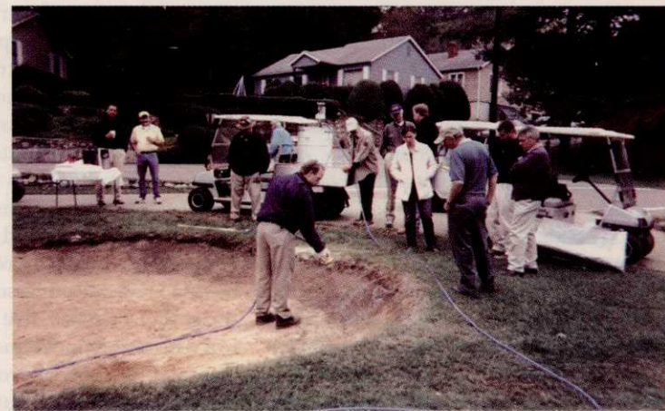
Co-inventor Tim Johnson installs Klingstone at Springhill Golf Club.
