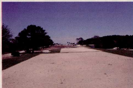
The full-scale renovation included new tees...
