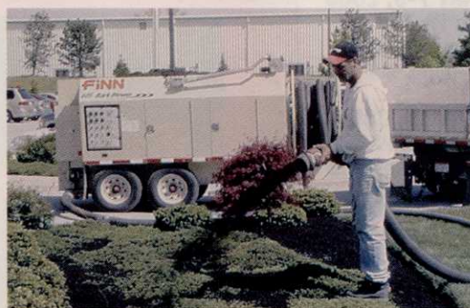
The unit can apply 15 to 30 cubic yards of material per hour.
