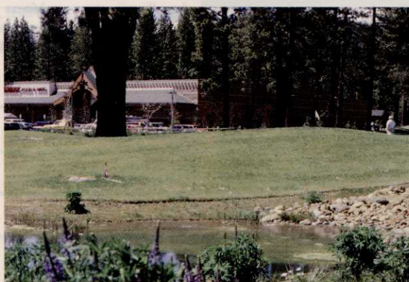
This drainage pond, located in front of a Safeway store under construction near a PGS client's golf course, solved major issues for all parties involved.
