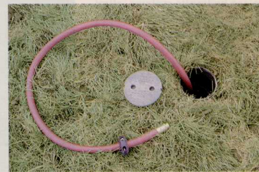
The pressurized, retractable hose is hidden underground.
